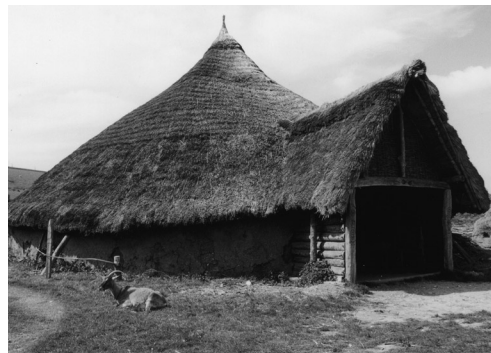
■ Figure 9.15 An Iron Age roundhouse at Butser Ancient Farm. 'Constructs' such as this have been immensely valuable in exploring many aspects of past buildings including roof shape, potential function, construction techniques and useful lifetime
