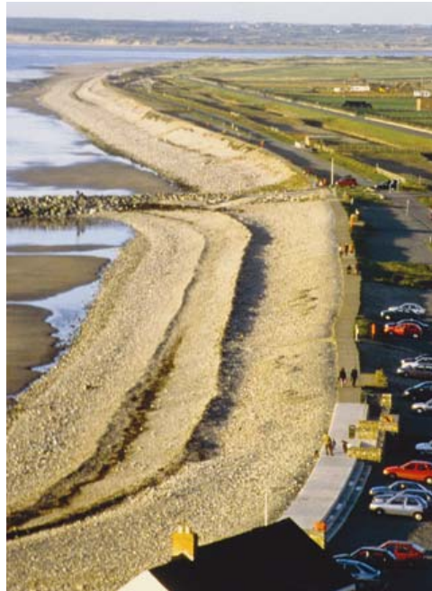
Plate 4 Semi-hard defences, in the form of a seawall fronted by constructed shingle banks and a transverse berm (mid-distance) protecting low-lying farmland and tourist infrastructure at Dinas Dinlle, on the Irish Sea coast of north-west Wales. A line of low dunes crests the shingle bank in the distance at the western end of the Menai Strait, across which can be seen the outline of Newborough Warren on Ynys Môn (Anglesey).
